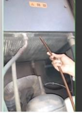
Clean all the fins of oil cooler by clean and dry air jet
